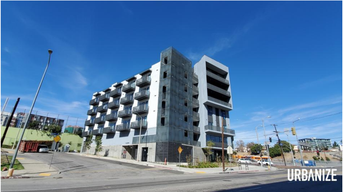
View of 1100 Temple Street looking northwest from Beaudry AvenueUrbanize LA
