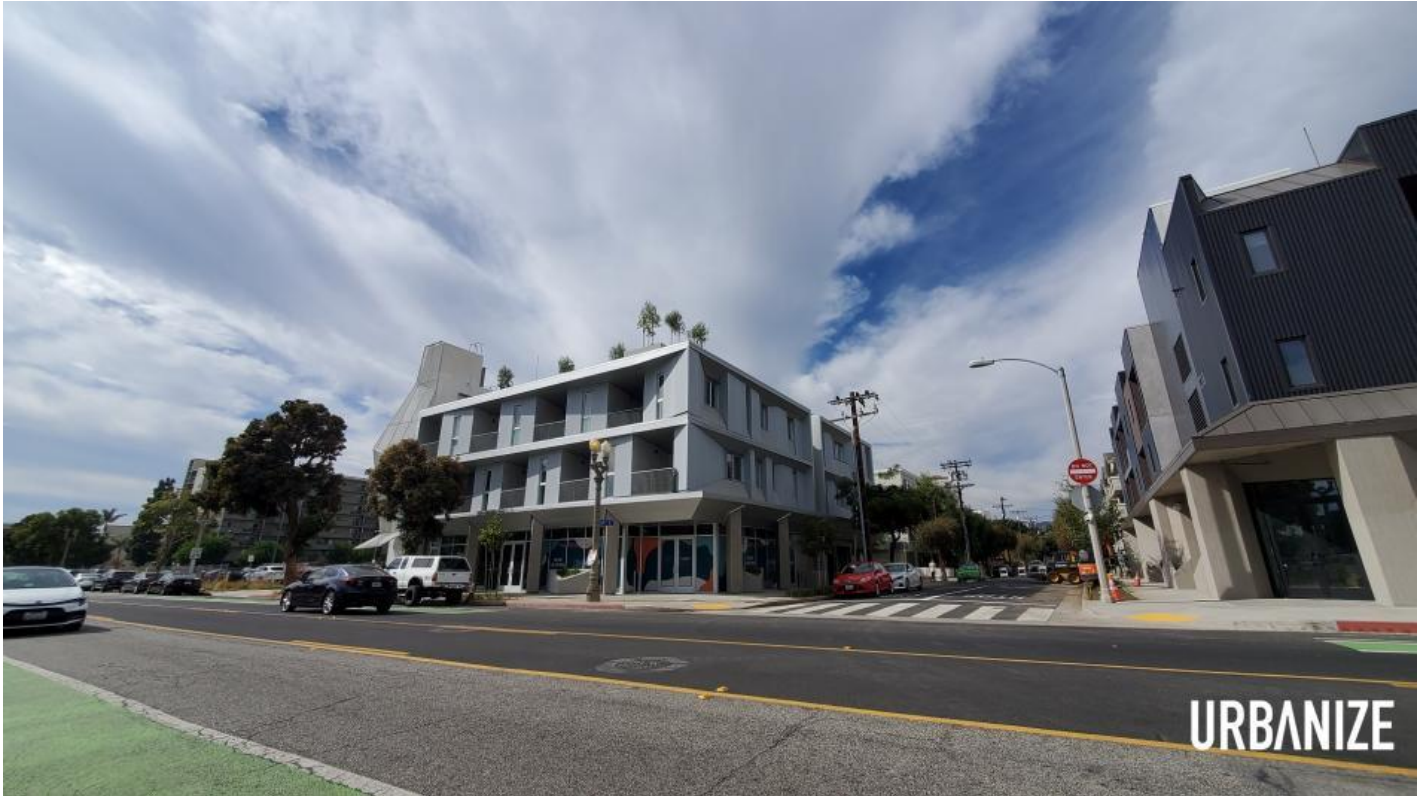
View of "The Charlie" from BroadwayUrbanize LA
