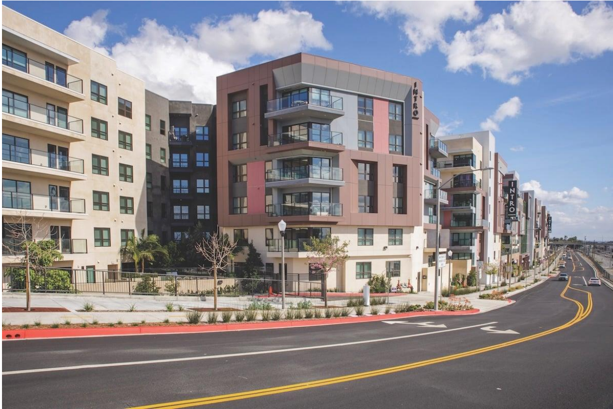
Exteriors of Intro, a mixed use development project in Burbank. (Photo by David Sprague)
